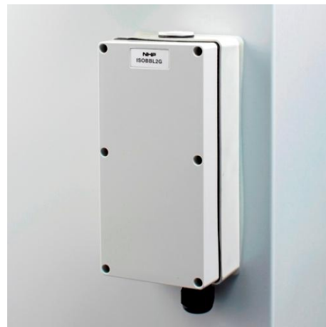
Electrical connection is via a junction box located on BlueGen and hardwired back to the electrical switchboard
