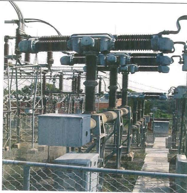
Figure 1 – Air-Blast Circuit Breaker
