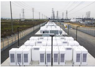
20MW / 80MWH 48 INVERTERS 396 POWERPACKS
