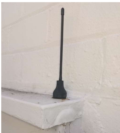
Photograph of the external antenna fitted to the author's smart meter
